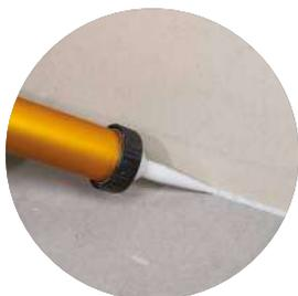
Sealing a through gap can produce an improvement of up to **+ 24 dB**.
